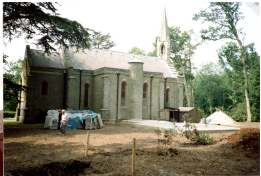
The footings in place
