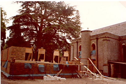
The building takes shape
