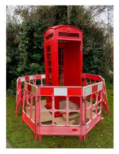
In October 2024 the work began to restore the metal frame of the box which had suffered many years of neglect. The old paint had to be tested for lead, then the rusty layers of paint were completely removed using a gas blow torch - a very challenging process undertaken by Mike Hansford. A pink primer and a red top coat were then applied.
